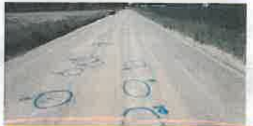
Figure B Example high-resolution, 36-mp image taken of unpaved roadway to automatically detect pothole density and severity, with project ground-truth markings shown
