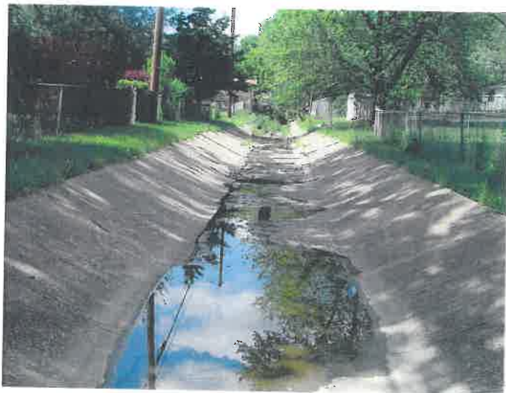
Failing Ditch Liner Between Fairlane and Holiday
