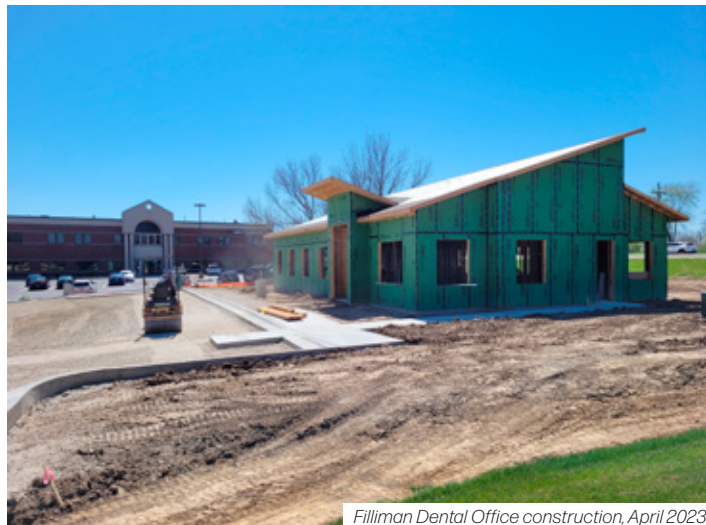
Filliman Dental Office construction, April 2023
