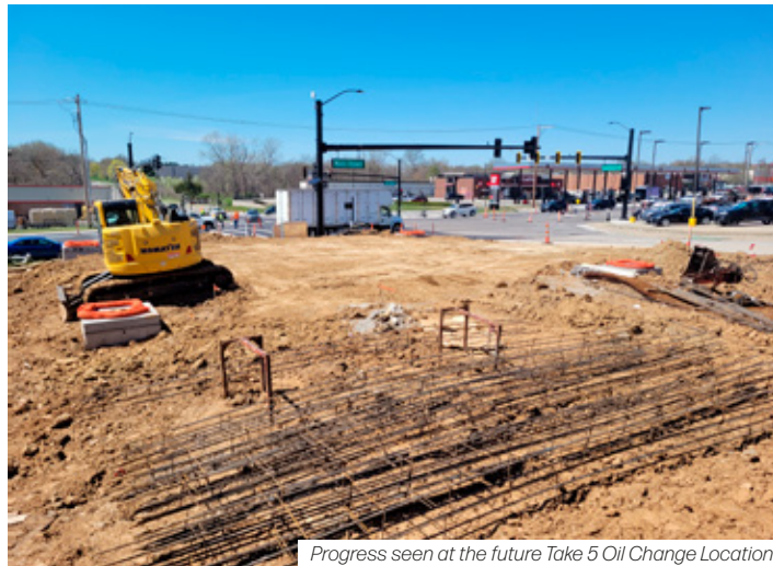
Progress seen at the future Take 5 Oil Change Location
