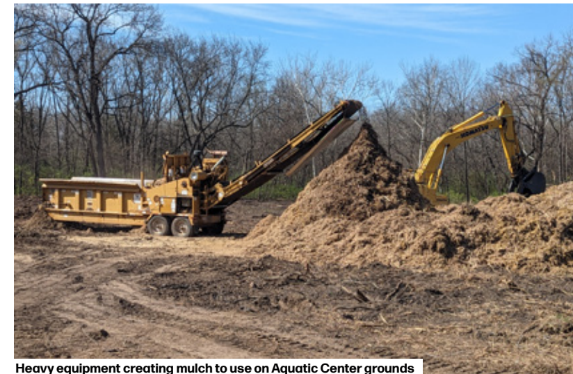
Heavy equipment creating mulch to use on Aquatic Center grounds
