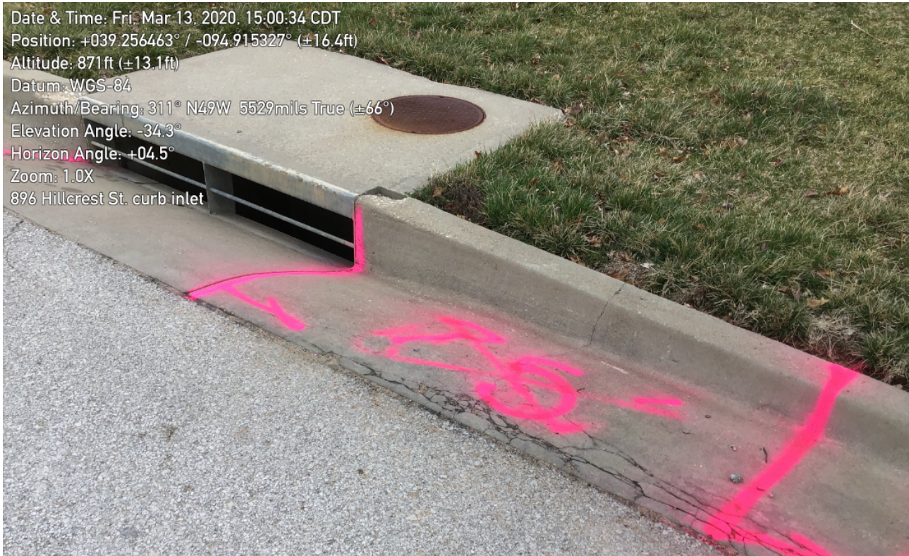
PHOTO-2 Curb failure example: SP-9 (6' min lengths, maximum varies)
