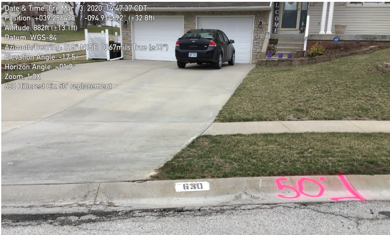
PHOTO-2 Curb failure example: SP-9 (6' min lengths, maximum varies)
