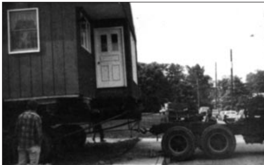
Figure 7-3 The journey to the new site begins.
