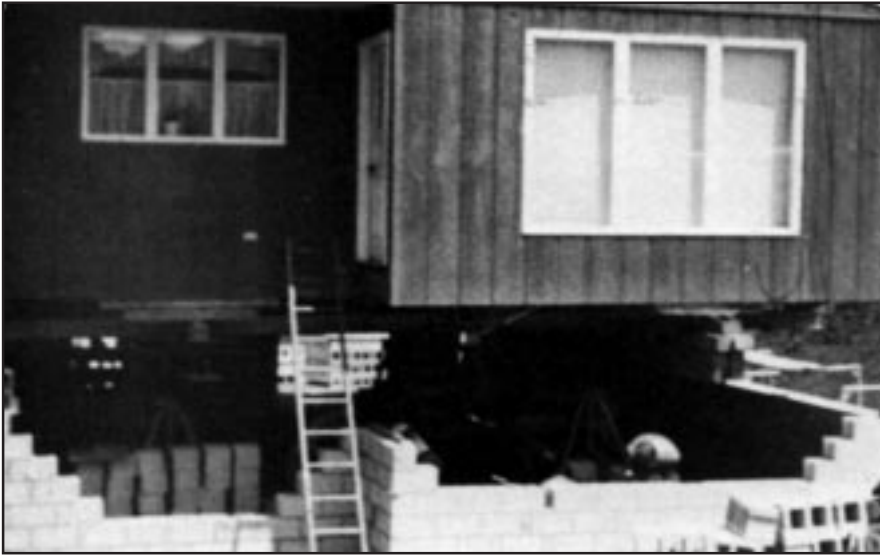
Figure 7-4 Once the house is raised, the foundation is completed.
